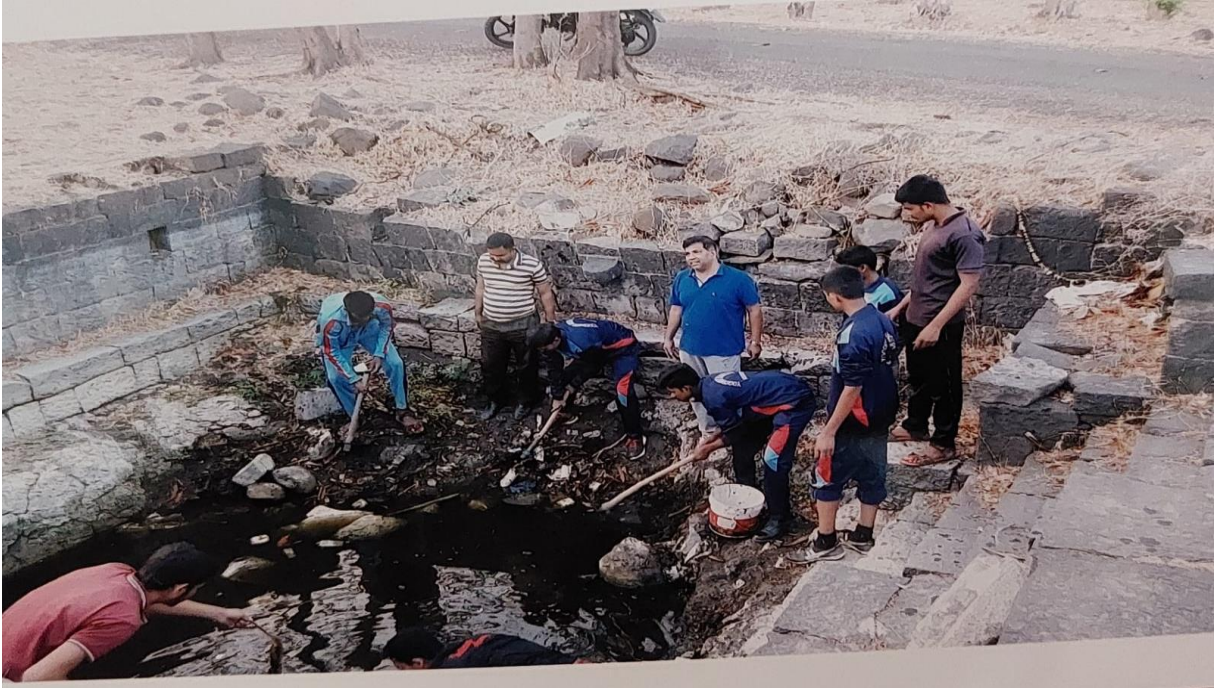
N.C.C. Cadets & Officers Excavating Mud from a Well at Dasopant, Ambajogai
