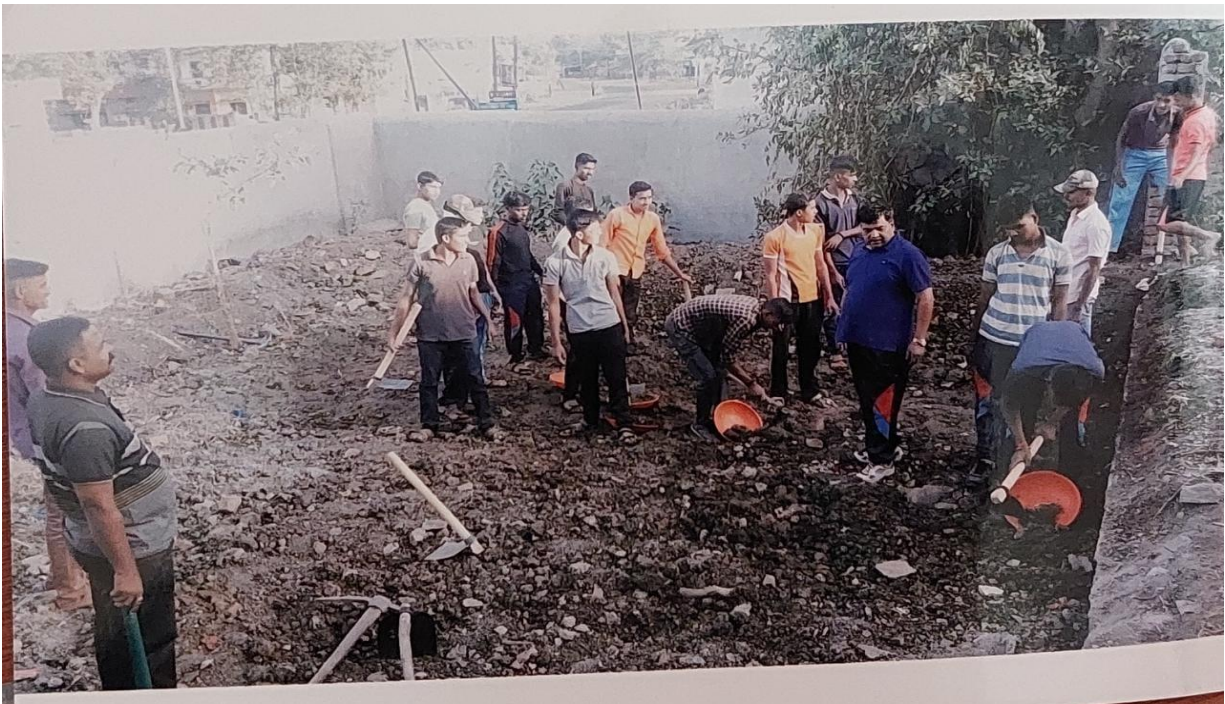
N.C.C. Cadets & Officers Excavating Mud from a Well at Hattikhana, Ambajogai
